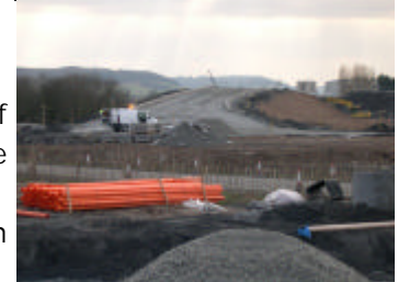
Work on Leominster Access Road, due for completion in August
